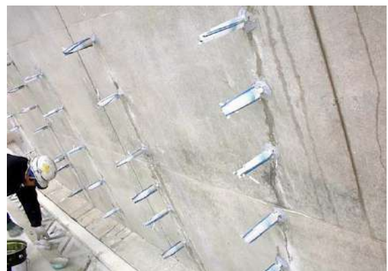
ひび割れ補修（低圧注入）状況：橋脚
